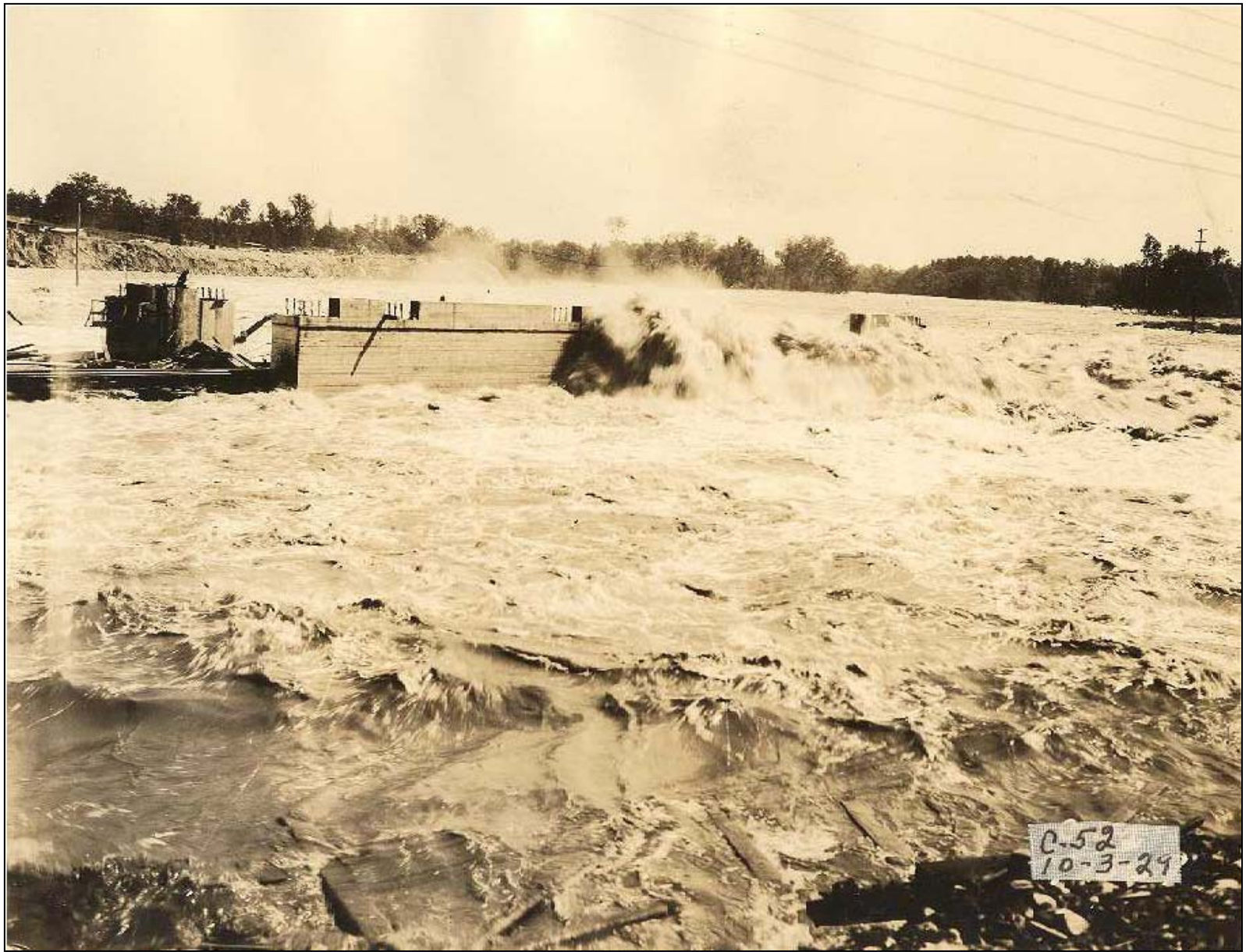
Powerhouse Foundation During Flood, October 1929
