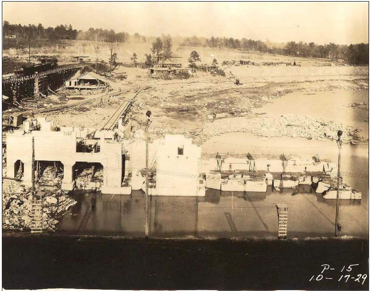
Powerhouse Foundation After Flood, October 1929
