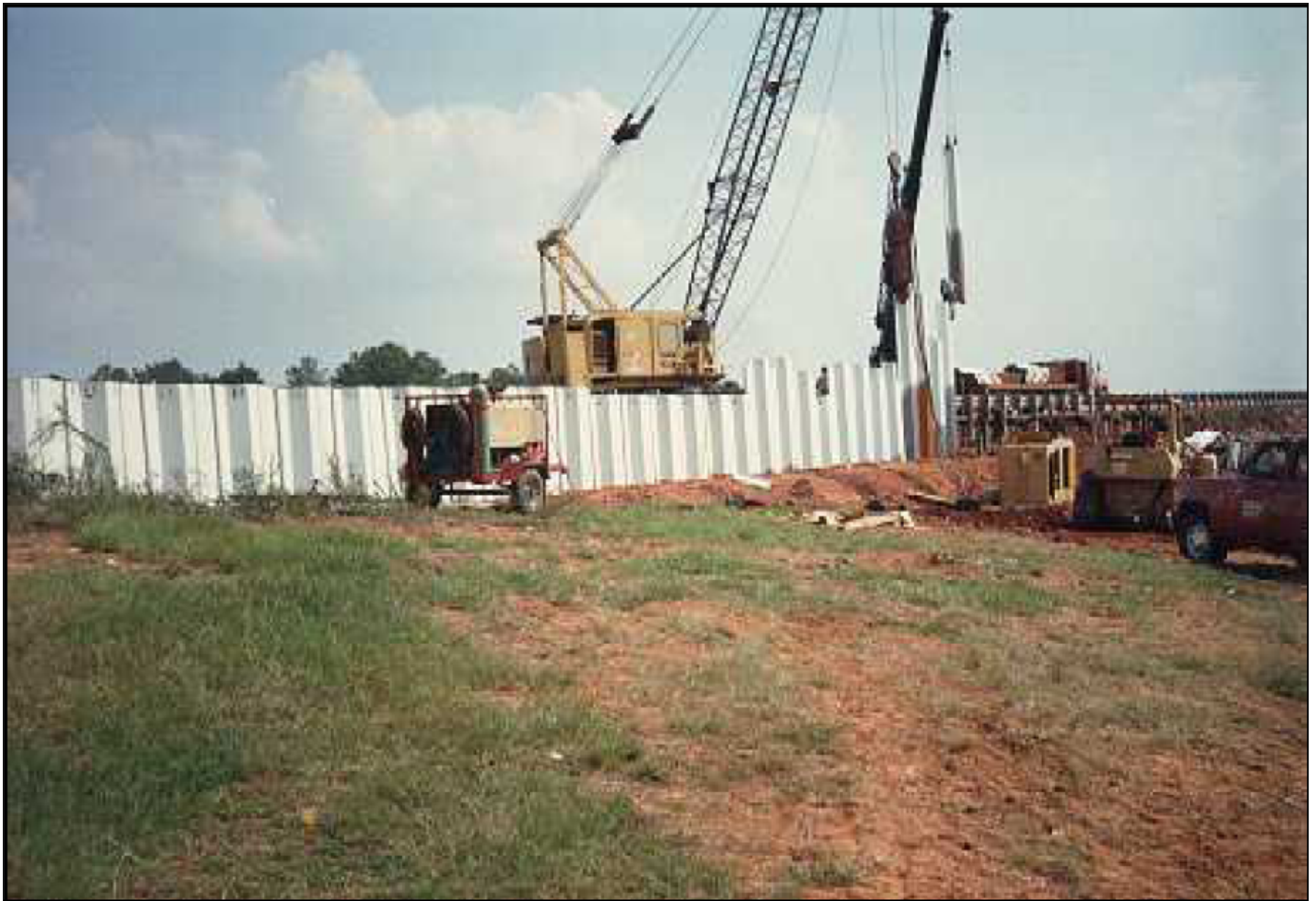
Sheet Pile Freeboard Wall Construction - 1990
